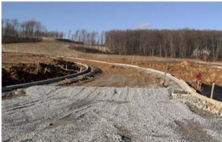
*Figure 5.7-2 Example of site development with extreme soil compaction on steep slope*
