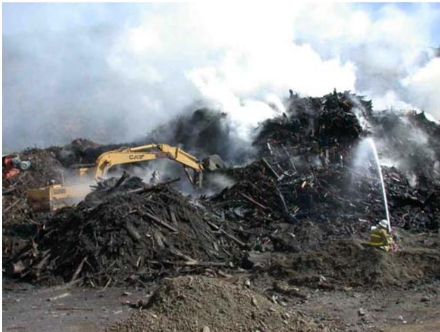
**Figure 4.6: LCGE material stockpiled in western Pennsylvania with no access roads between the piles. Equipment cannot efficiently access the fire area in this case.**
